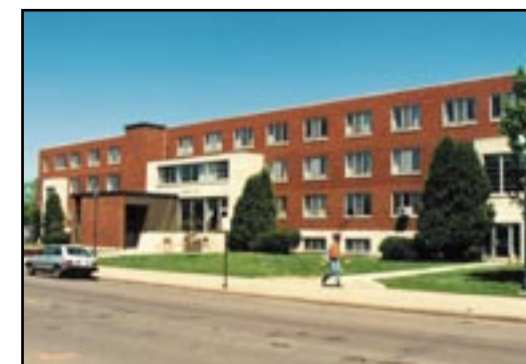
Sundquist Hall to be razed (Demolition 2009-11 GPR)
